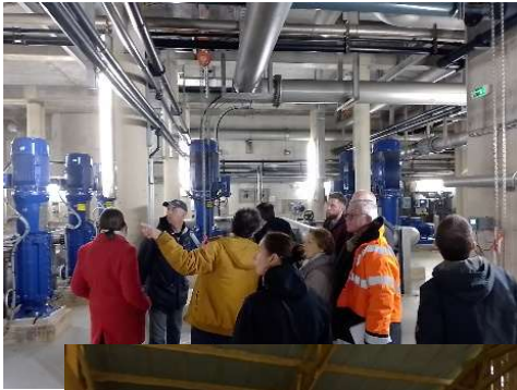
Usine eau potable - Châteaubourg
